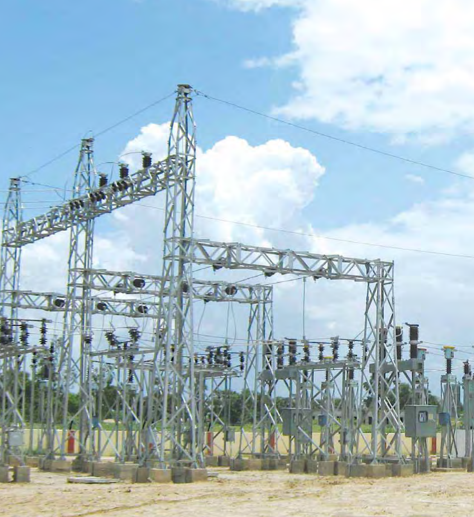
33/11 kV Power Substation at Nardiganj, Bihar under RGGVY (Rajiv Gandhi Grameen Vidyutikaran Yojana) scheme
