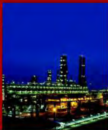
✓ Industrial Power Distribution
