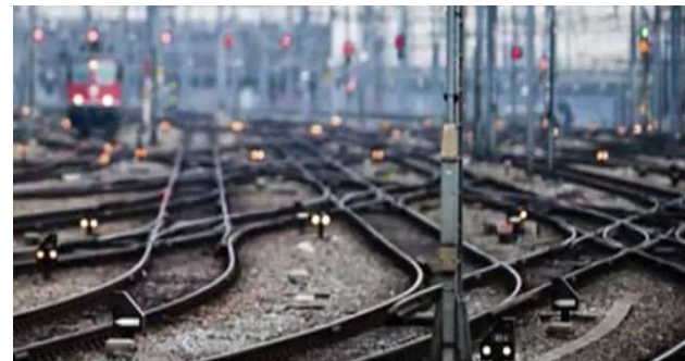
Civil & Track works
